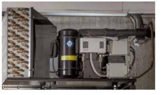
**(2)** The **climate equipment** assembly dispenses heat generated in the wine cellar. It is always installed outside of the wine cellar and models are offered according to the particular endemic conditions.
