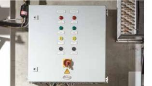
**(3)** The third component is the **electronic module** which is installed close to the climate unit.
